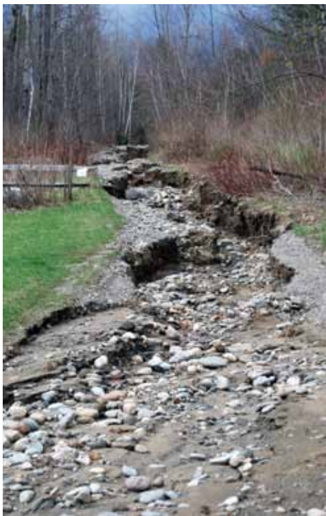
The destroyed Bolton Quarry driveway shortly after the April 26 flood.
